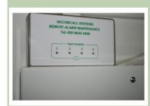
Securicall have developed a sophisticated device called a Remote Alarm Maintenance control unit (RM201), which is installed in your premises adjacent to the main intruder alarm control panel. By appointment, this enables us to do
